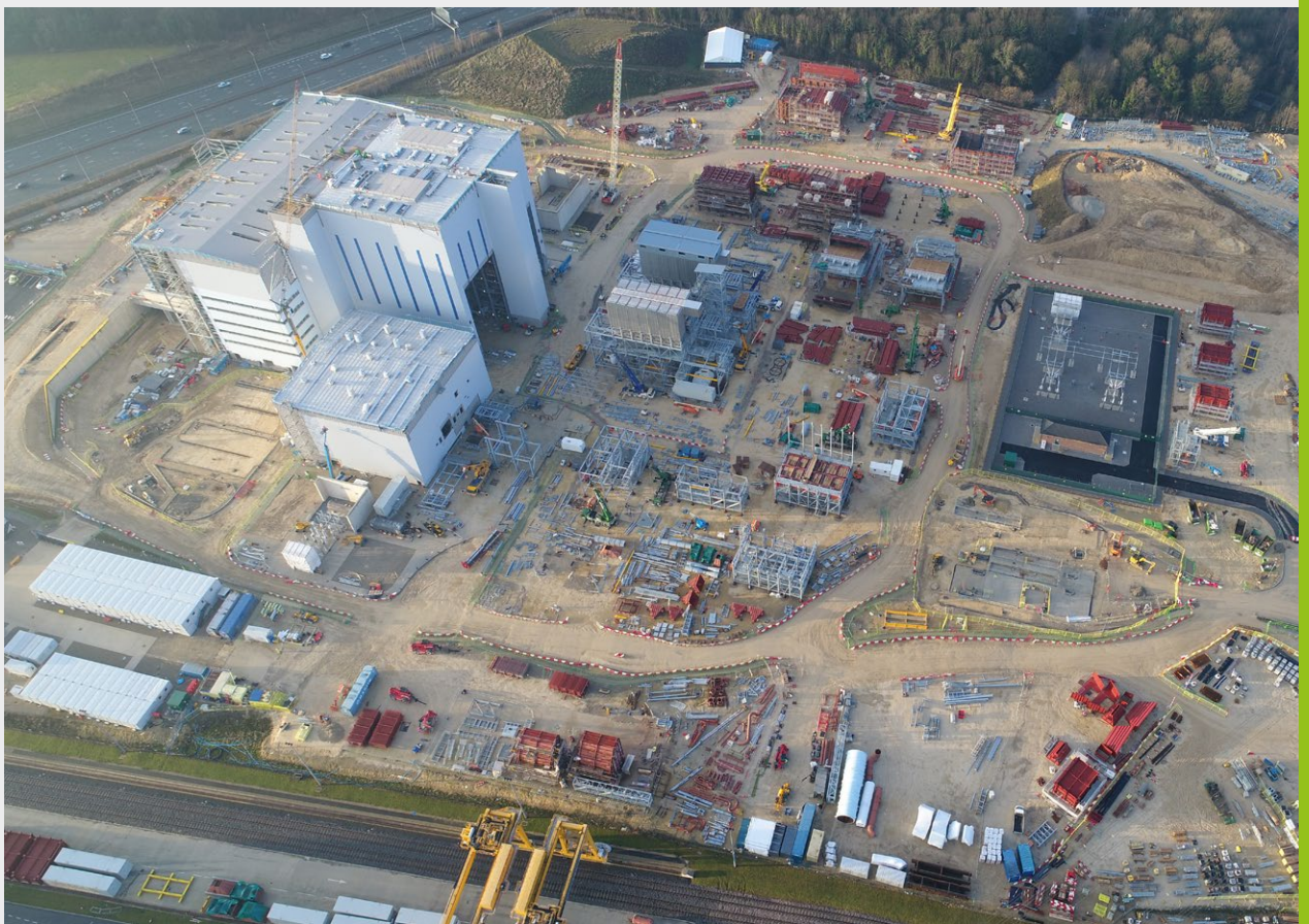
WtE plant under construction in Ferrybridge, UK
