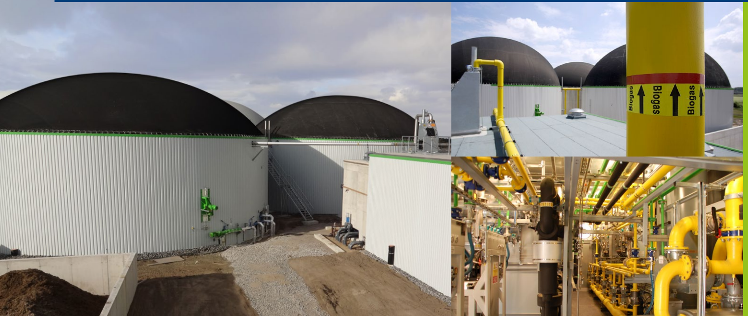
Biogas plant with gas upgrading unit for gas grid injection
