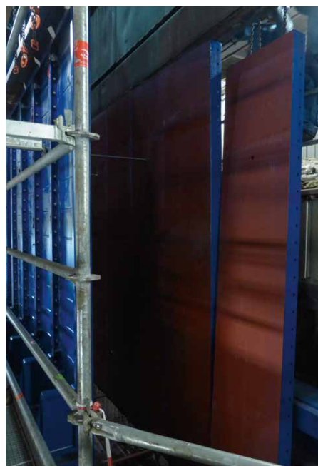
EfW plant Zistersdorf (l) – erection of the modules; EfW plant Zorbau L2 (r) – inspection of the inner surfaces (cladding with alloy and S235JR) after 2 years' running time
