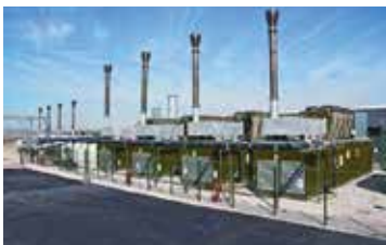
At ITC's existing landfill gas site in Ankara it uses the heat from the engines in a greenhouse to grow tomatoes and strawberries.
